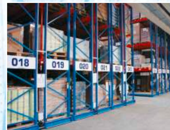
Piping material warehouse
